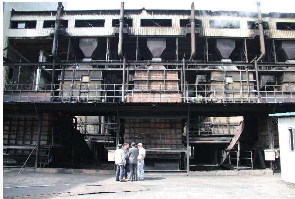
Semi-coke plant in Shaanxi province, China
