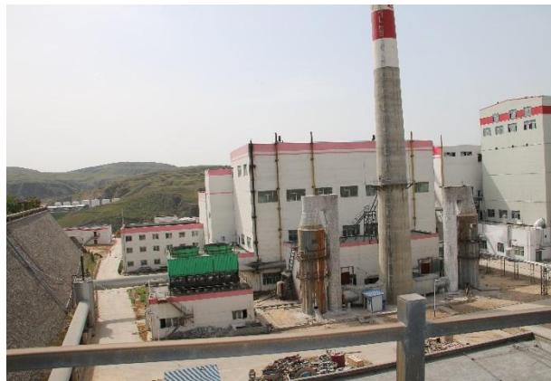
Crude gas power plant
